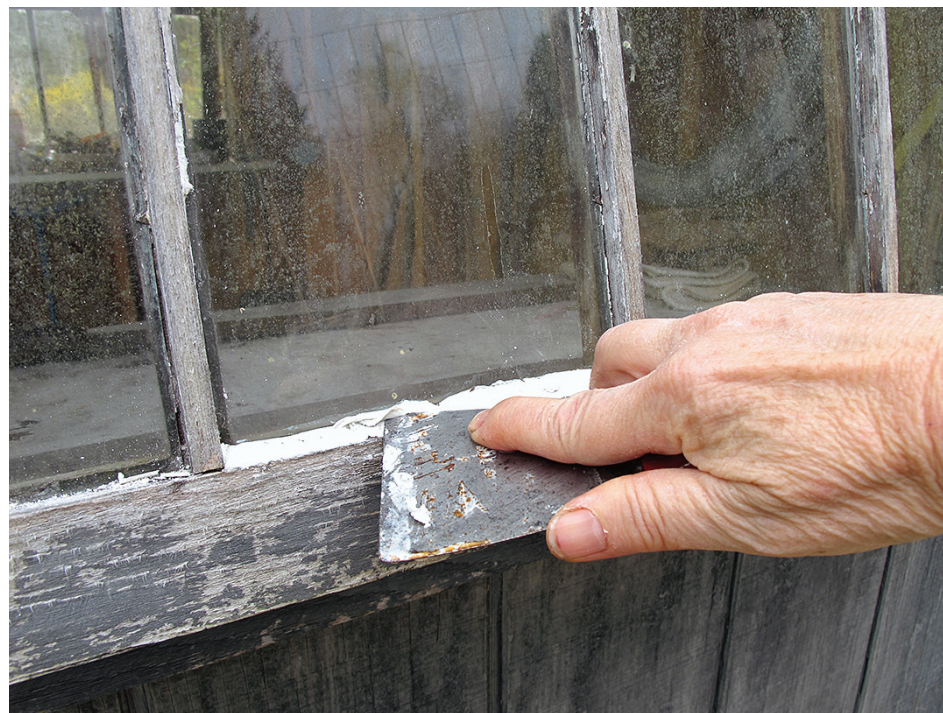
The worm is smoothed with mineral spirits on a knife.
