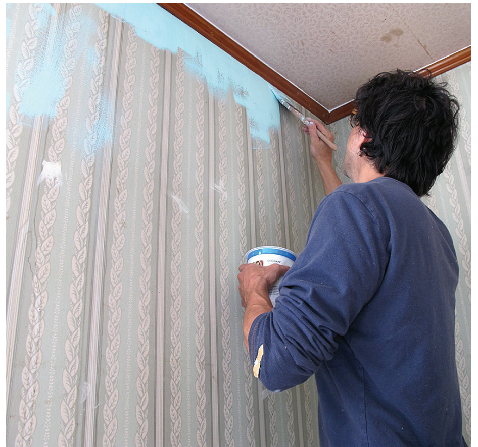
After careful prep work to make sure it stayed flat, the wallpaper was painted over.
