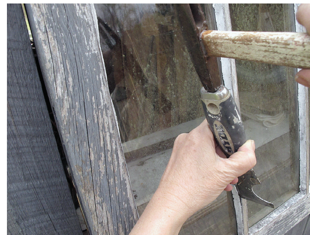
A small hammer and 5-in-1 are used to remove putty.
