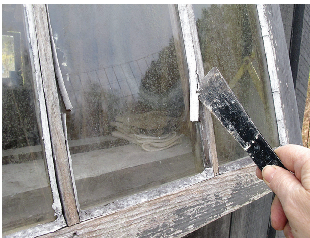
Old glazing is removed using a mini-flat bar.
